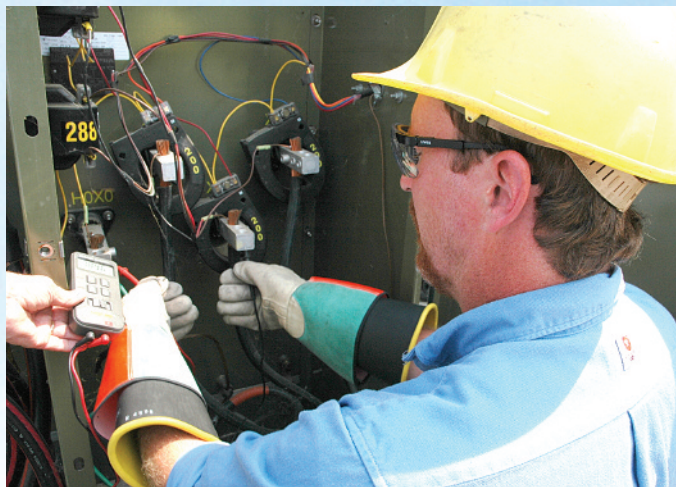
POWER PARTICULARS: Terry Hutchison, director of engineering and technical services at Valley REC, tests the photovoltaic system at the station to see if equipment responds properly to power grid fluctuations.
