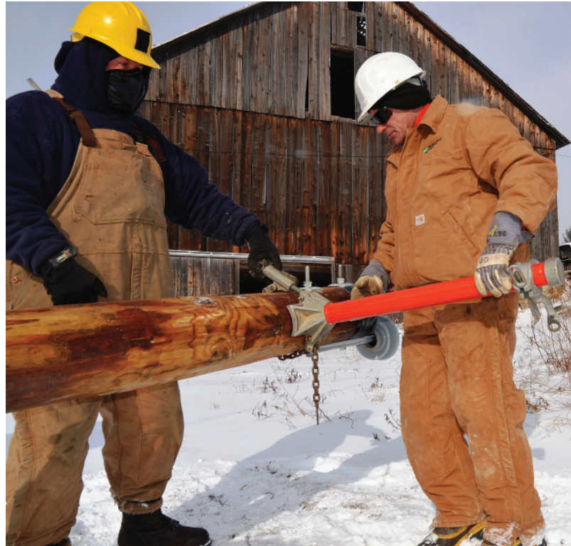
Far left: Braving a 5-degree morning, journeyman linemen Bill Bogel, left, Bill Kreider and Greg Dilling, crew chief, prepare to set a new pole in Juniata Township, Blair County, as Justin Berrier operates the auger. At left: A small herd of buffalo near Blue Knob watches Berrier operate the track digger. Above: Bogel, left, and Dilling place a temporary line holder, called a layout arm, on a pole. Below: Work is progressing on a project to replace aging poles and string new wire near Perulack, Juniata County. (Photos by Doug Roles)
