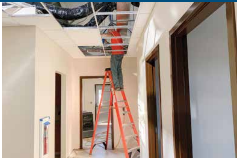
RUNNING CABLES : Valley’s Information Technology Manager, Max Hetrick, running ethernet cables during the construction phase of the new Martinsburg District office.
