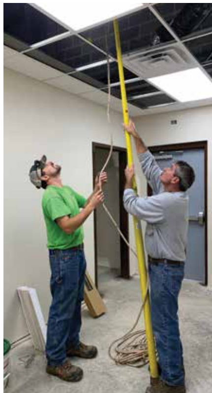
HARD AT WORK: Valley linemen Trevor Eichelberger, left, and Greg Dilling brace the lighting system in the new office building.
