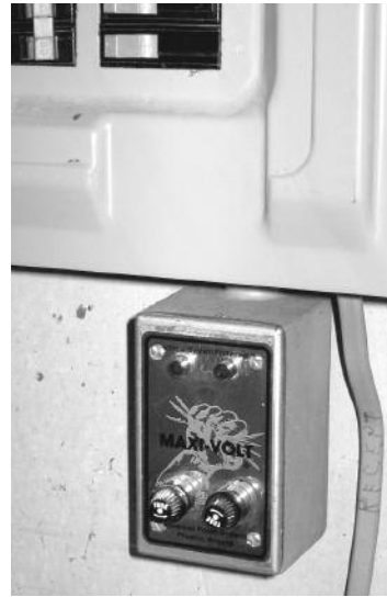
SURGE SAVIOR: This particular whole house surge suppressor is mounted beneath a circuit breaker panel. Source: James Dulley
