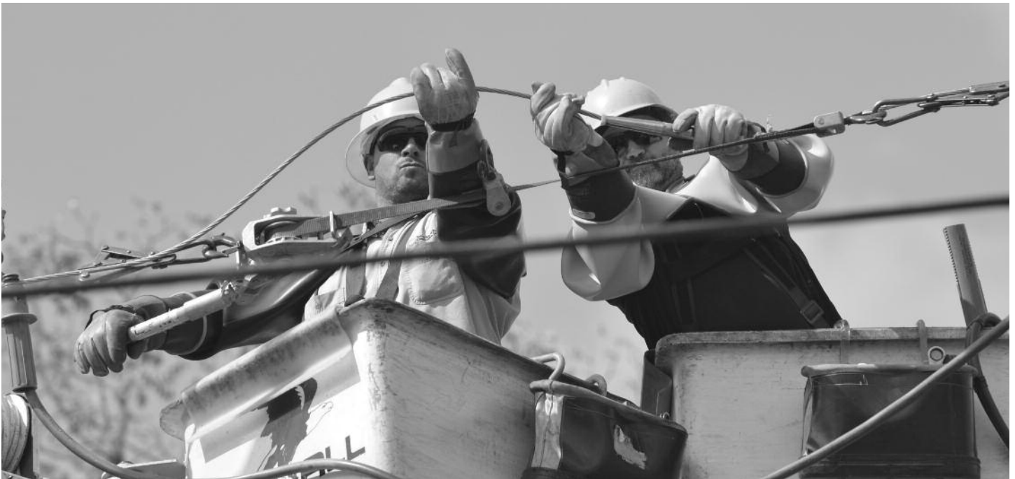
Valley REC linemen Jason Wilson (left) and Mike Williams make a live-wire connection. (Photo by Doug Roles)
