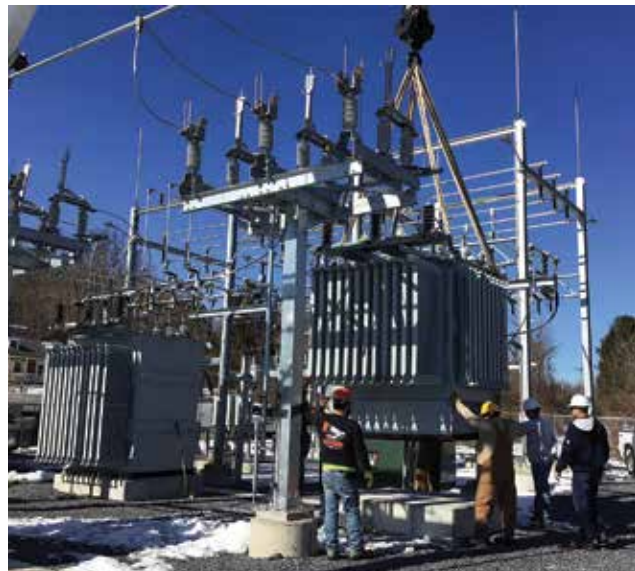
A Greiner Industries crane crew lowers a spare transformer back into Valley REC's new Path Valley Substation Feb. 24, 2021. The unit had been removed for repairs due to a manufacturer's defect. The substation in Franklin County serves members in the Fort Loudon and Cowans Gap areas. Photos by Doug Roles
