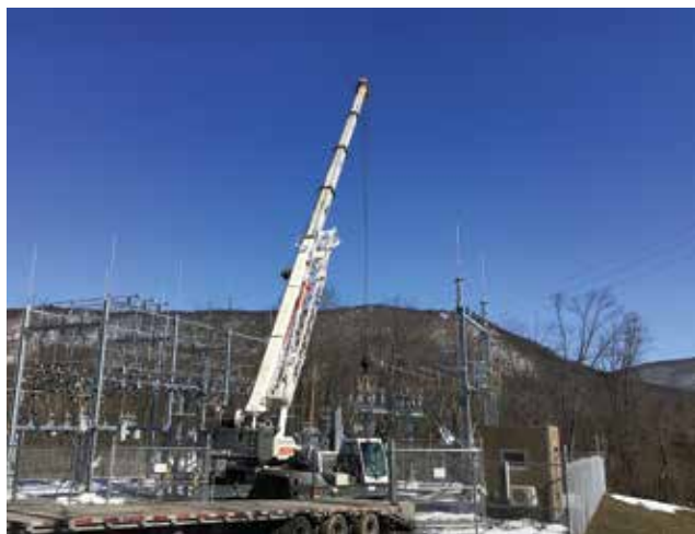
A Greiner Industries crane crew lowers a spare transformer back into Valley REC's new Path Valley Substation Feb. 24, 2021. The unit had been removed for repairs due to a manufacturer's defect. The substation in Franklin County serves members in the Fort Loudon and Cowans Gap areas. Photos by Doug Roles
