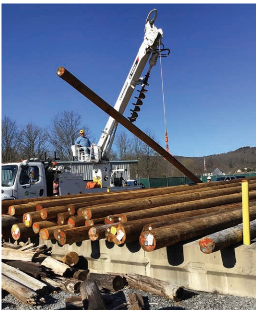
HEAVY LIFT: A lineworker lifts a utility pole from the pole yard with a digger truck.
