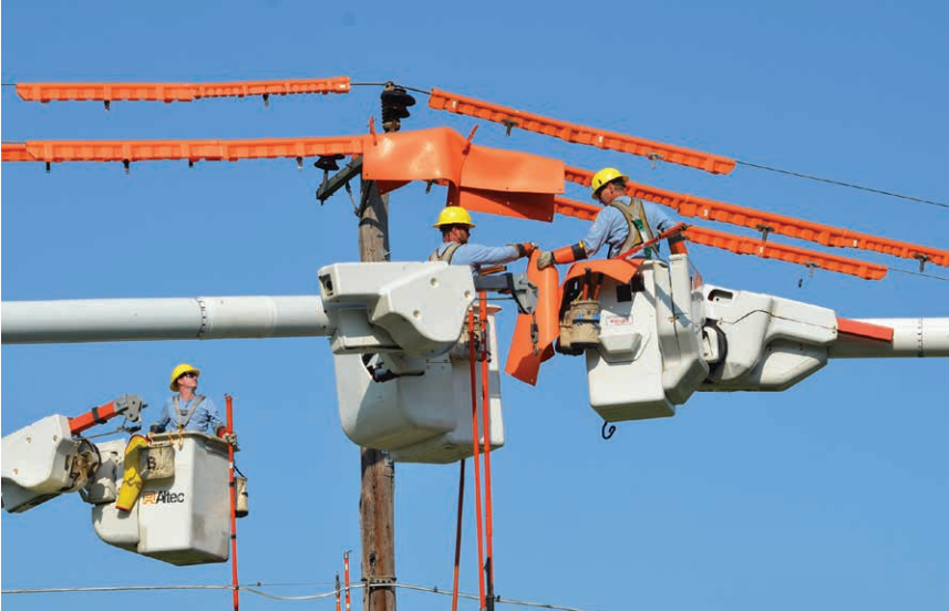
ON THE JOB: Our lineworkers have all kinds of tasks that keep their careers interesting. They wouldn't have it any other way. Clockwise, from top left: From left, Cody Accord, Dane Diehl and Ryan Dodson place rubber blankets over energized power lines near Blue Knob during annual on-the-job training in mid-September. Top right: Diehl finds himself in a maze of rhododendrons in North Carolina after Hurricane Helene. Valley REC crews were among those to help restore power after the storm. Bottom right: From left, Curtis Starr, Jason Wilson, Diehl and Seth Glover pause for an early morning photo Oct. 8 before leaving the Shade Gap office to assist with power restoration efforts in North Carolina. Bottom center: Logan Booher takes time to answer electric safety questions from young attendees at Mapleton Volunteer Fire Company's open house Oct. 10. Bottom left: Matt Fish, left, and Riley Price demonstrate that a leather glove offers no protection against high voltage during a hot line demo at Mapleton Volunteer Fire Company's open house.
