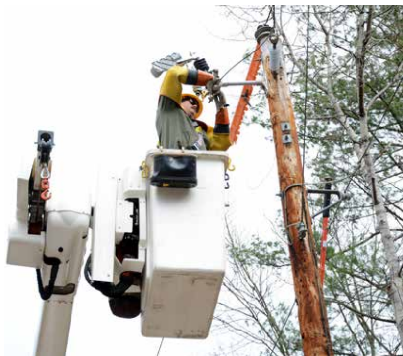
FINISHING THE JOB: Valley Rural Electric Cooperative Journeyman Lineman Logan Booher installs a cut-out fuse on a pole in Tuscarora Township, Juniata County, in November. The installation was the final one in the Shade Gap service district and was part of a multi-year sectionalizing effort.
