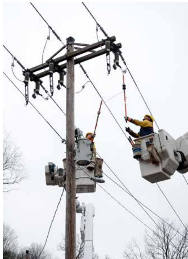
LINE TEST: Valley Rural Electric Cooperative Linemen Cody Acord, left, and Dane Diehl use a phasing tester to verify line voltage before re-energizing the Puzzletown substation in November.
