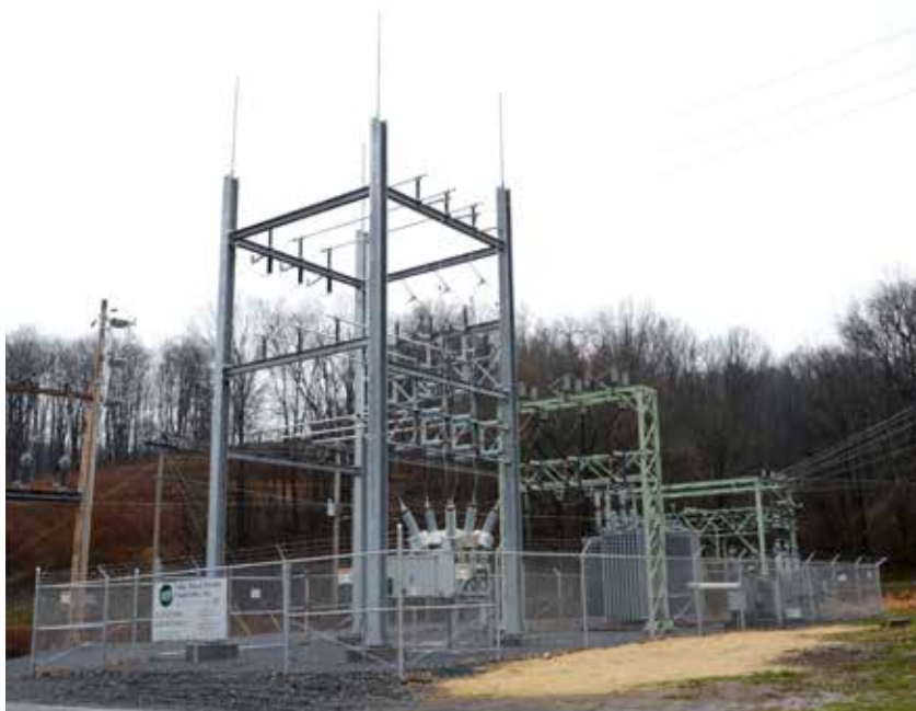
SUBSTATION REPLACEMENT: Through the fall of 2025, the Puzzletown substation in Blair County was a busy place. Co-op personnel and contracted crews replaced a high-voltage substation breaker and erected a new metal framework in place of an aging wooden structure. The upgraded substation, left, was re-energized Nov. 19.
