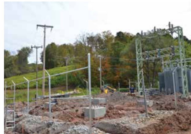
SUBSTATION REPLACEMENT: Through the fall of 2025, the Puzzletown substation in Blair County was a busy place. Co-op personnel and contracted crews replaced a high-voltage substation breaker and erected a new metal framework in place of an aging wooden structure. The upgraded substation, left, was re-energized Nov. 19.
